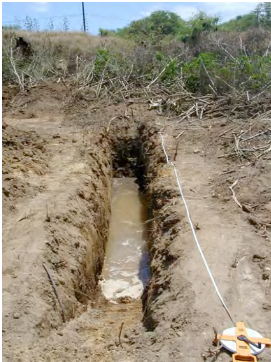
PHOTO 18 Trench C-3, view north.
