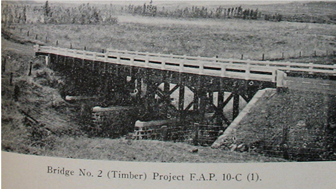
Fig. 2: Photograph of Bridge No. 2, which was built at the same time and following same standard plans as Bridges 3 & 3A. Superintendent of Public Works Report for 1940.
