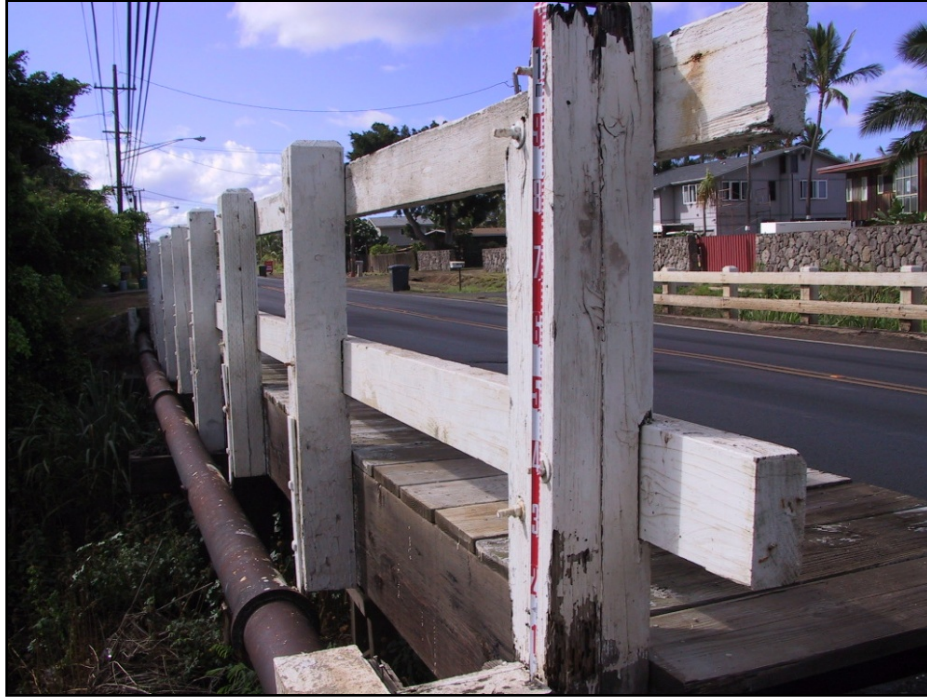
Figure 20. Photograph of SIHP # 50-80-07-6822, wooden guardrail and metal pipe; view southeast/east
