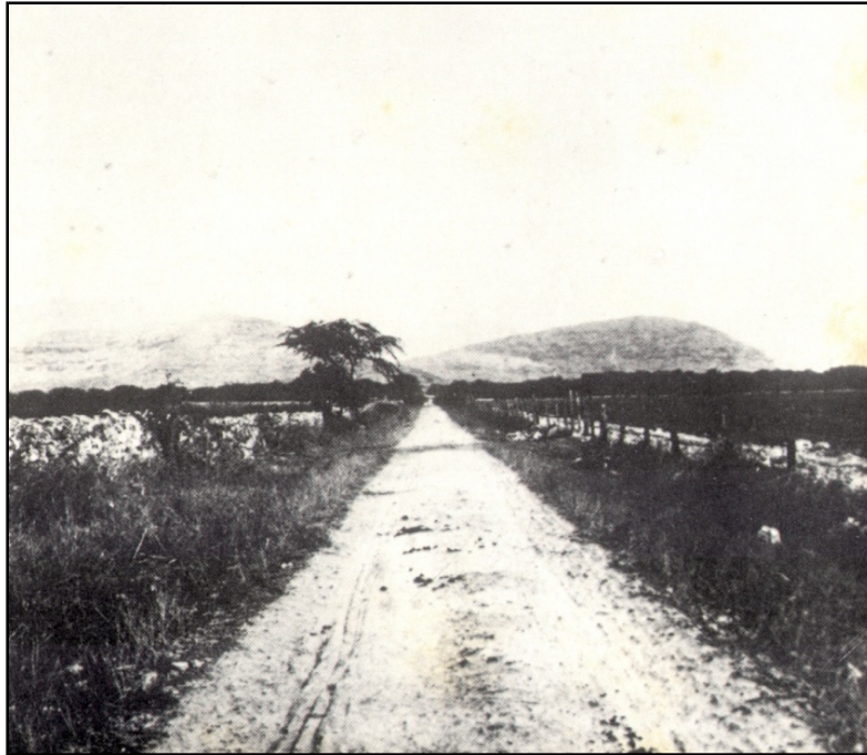
Figure 7. Photograph of the old Waianae Road (McGrath et al. 1973:51)
