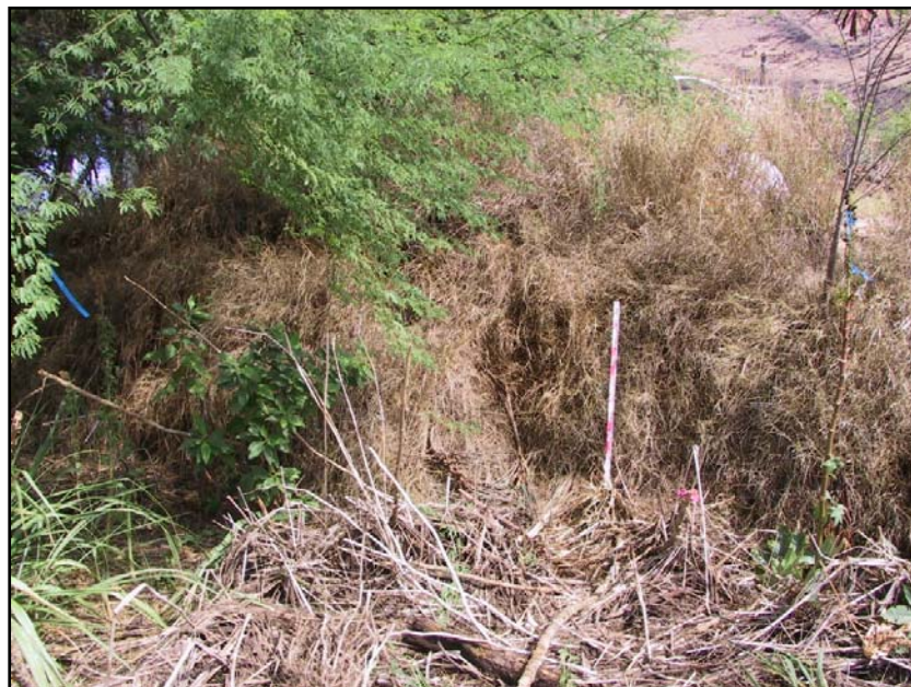
Figure 37. Photograph of the northern abutment of Feature B, SIHP # 50-80-12-9714; view north
