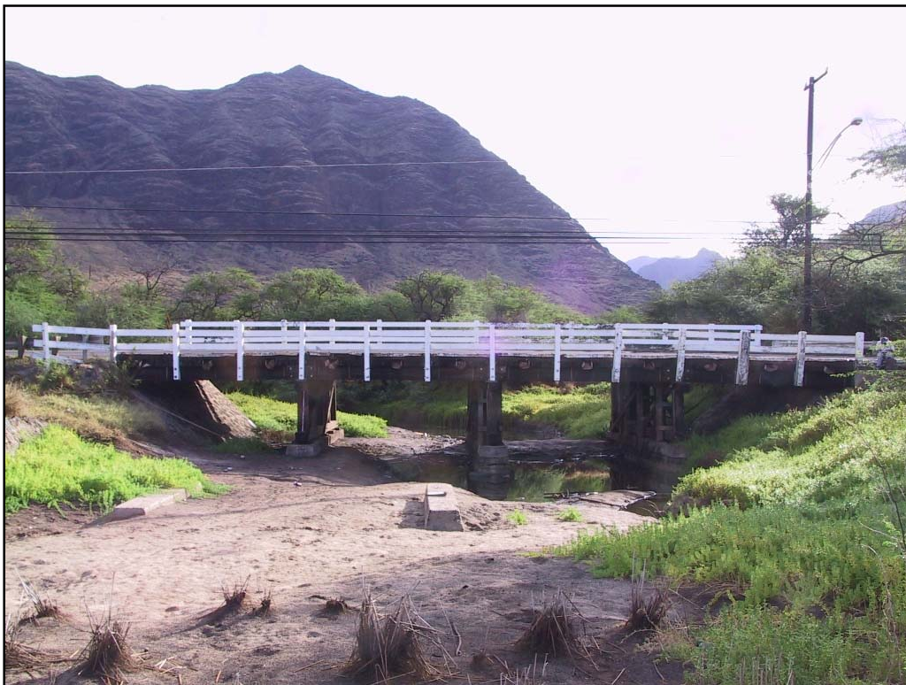
Figure 29. Photograph of SHIP # 50-80-07-6823, view to the northeast
