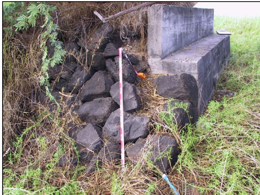
Figure 39. Photograph of the southern abutment of Feature C, SIHP # 50-80-12-9714; view west
