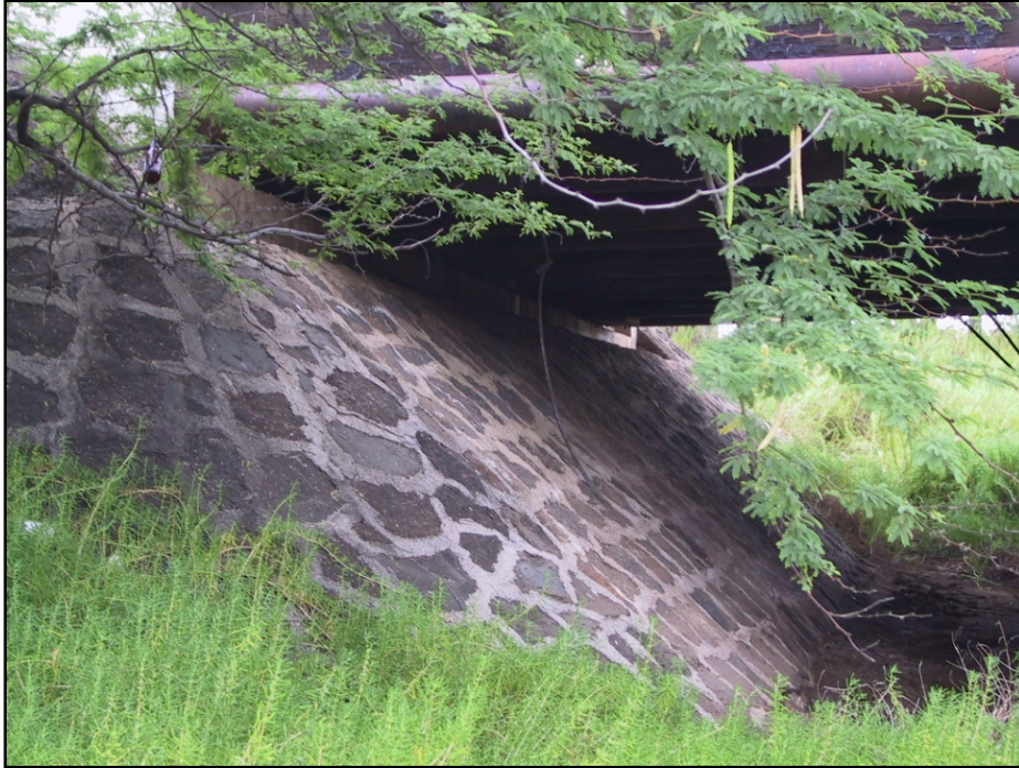
Figure 25. Photograph of SHIP # 50-80-07-6823, blue rock and mortar abutment; view west
