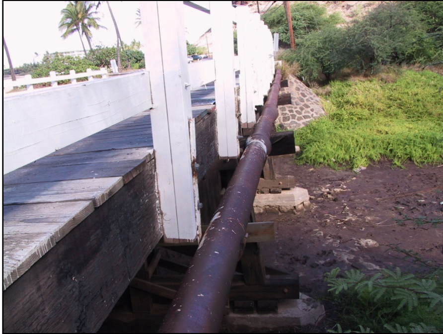
Figure 27. Photograph of SHIP # 50-80-07-6823, wooden guardrail and metal pipe; view northwest
