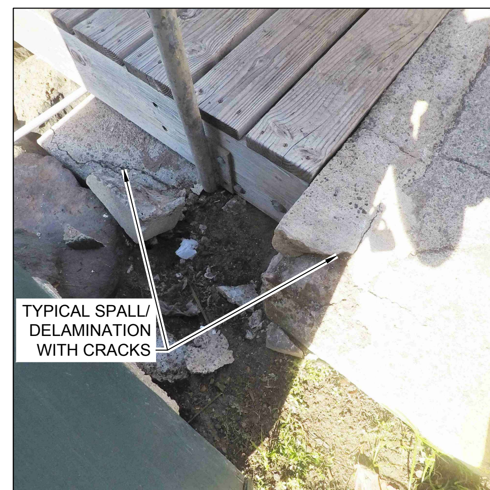
PHOTO - TYPICAL LANDING CONCRETE DEFECTS SCALE: NTS
