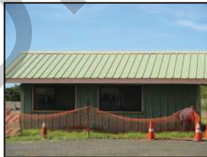
Site Office Building November 2019
