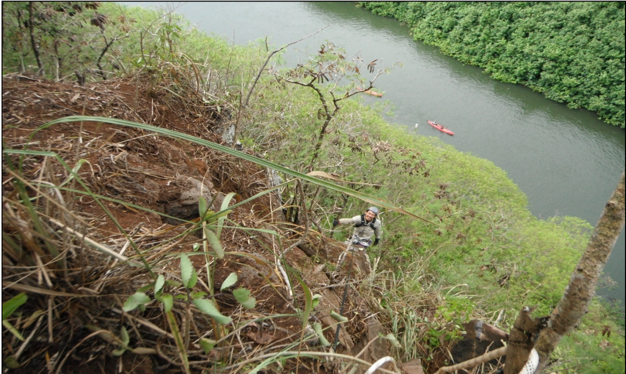
Wailua River from Rockfall Location 1; view to south down the cliff.
