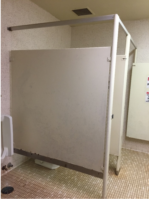
Typical toilet partitions to be replaced. Not shown, urinal screen
