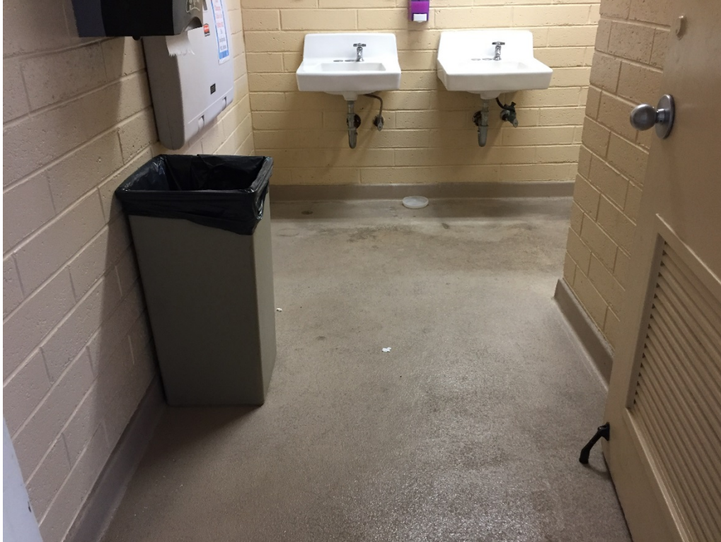
Typical entry to the restrooms
