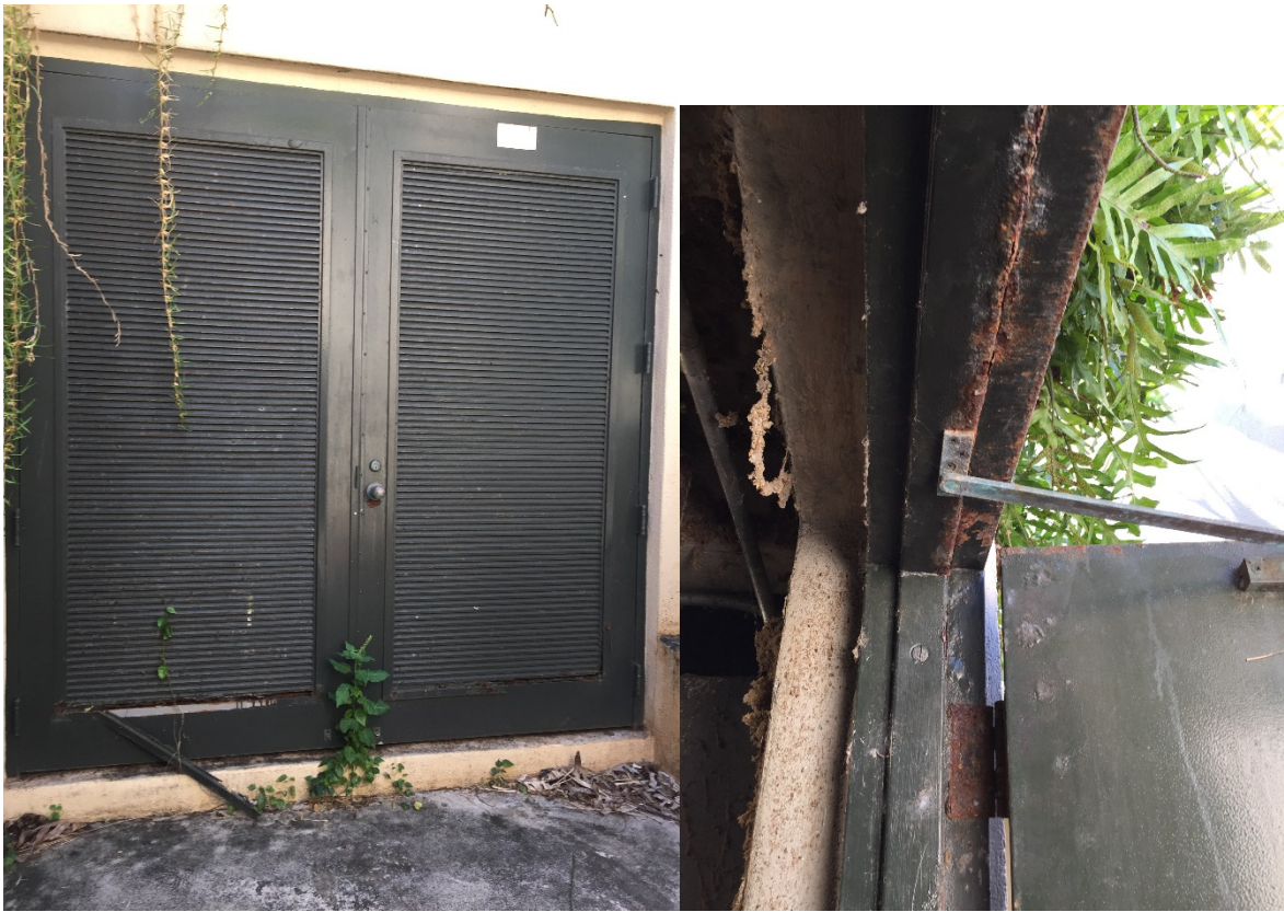
Transformer vault room door and mechanical room door frame.
