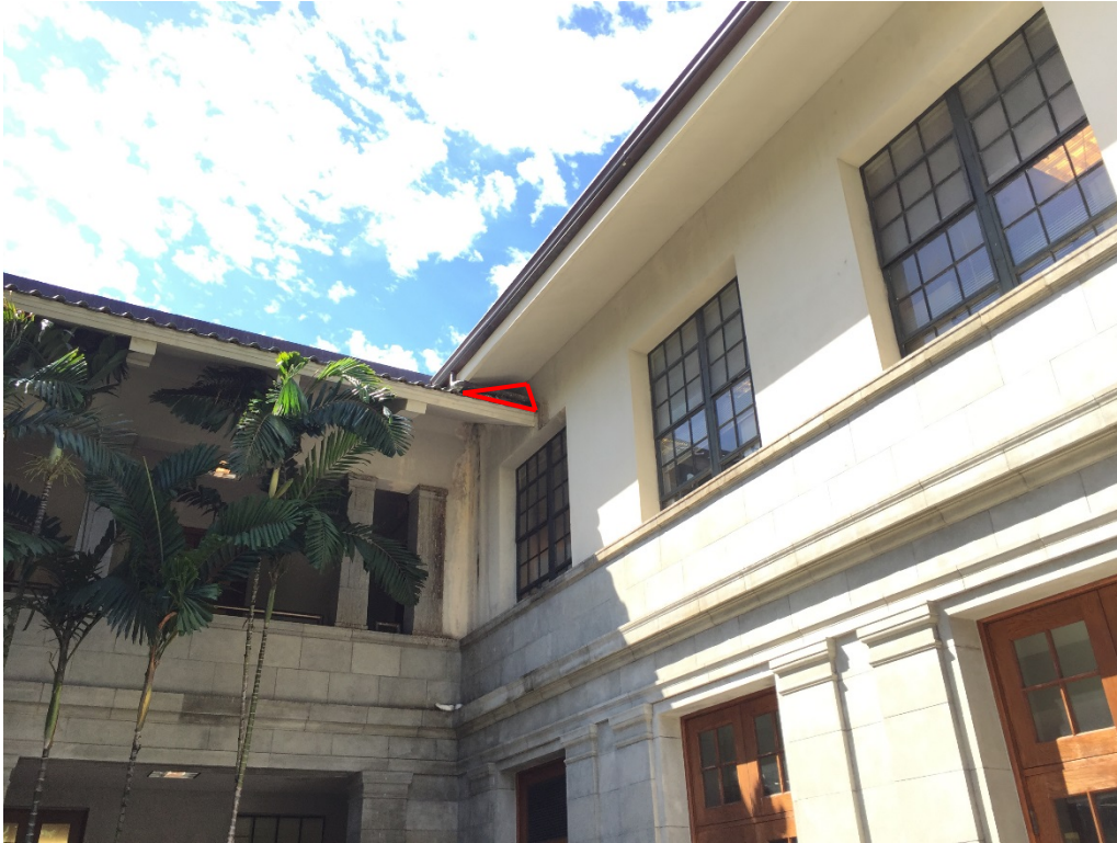
Courtyard area where bird netting to be installed (outlined in red).
