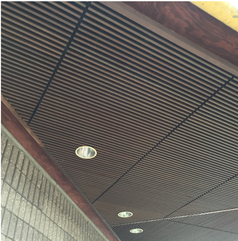
Wood soffit at drive-thru book drop
