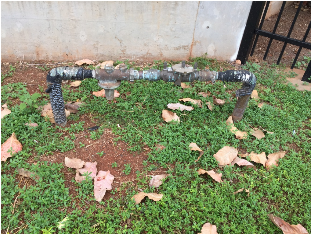
One of two BFPAs to receive enclosure. Approximate dimensions: 47"W x 8"H.
