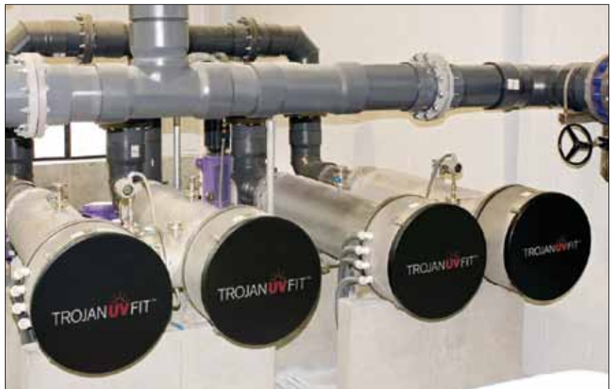
Reactors can be installed in parallel or in series for increased design and installation flexibility.
