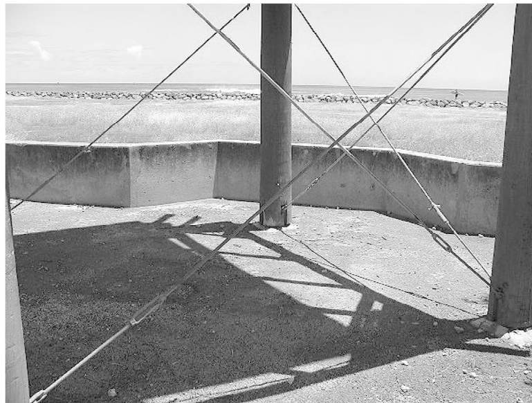
Battery Harbor, Emplacement No. 1, looking south.
