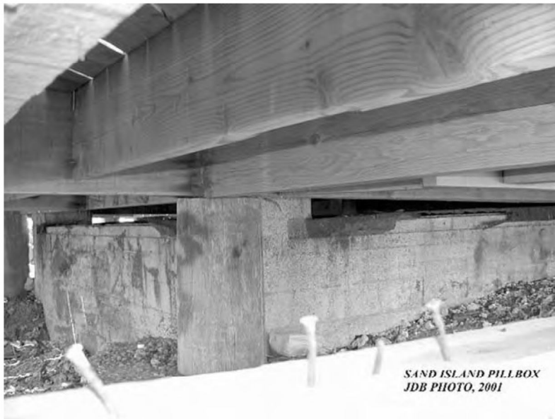
Observation slits on north and east walls of 1934 machine gun pillbox.
